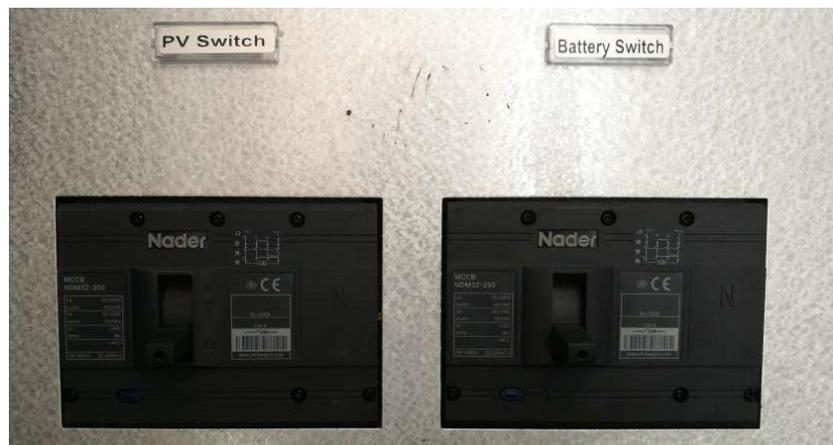
Figure 5.3 PV switch and battery switch in switch-off status
