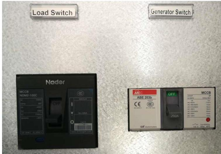
Figure 5.5 Load switch and diesel switch in switch-off status
